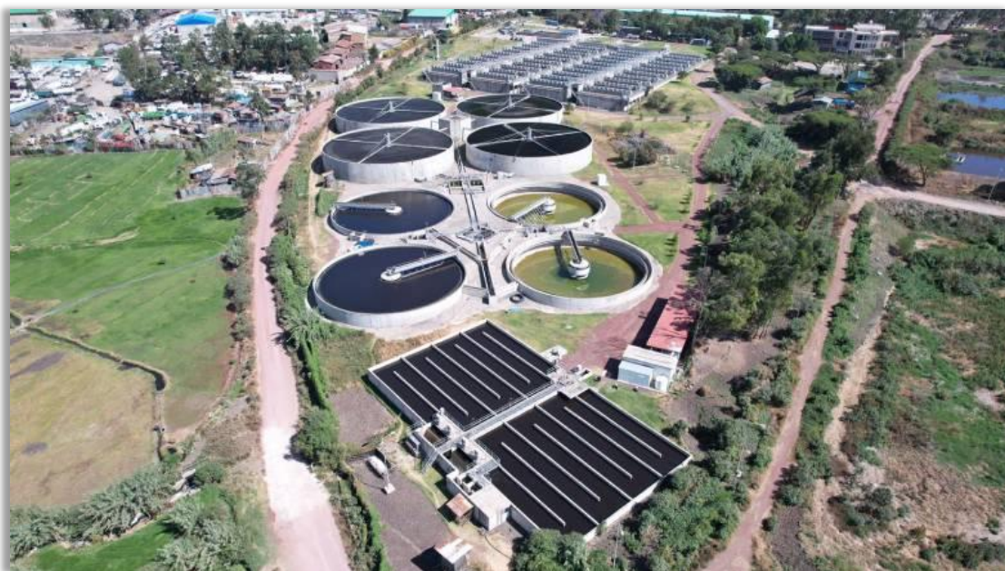
Kaliti wastewater treatment plant (upgraded & modernized, treats up to 100,000 cubic meters per day, and repurposes water for irrigation)
