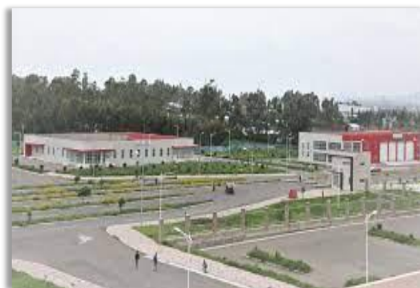
Kilinto industrial park
