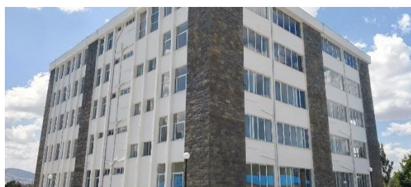
The newly constructed Akaki Health Center in Akaki Kaliti Sub-city
